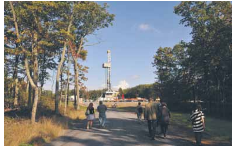
Soon, more trees will be cut down along the road, a new clearing will be made, the road, the pipeline and the water supply will advance a few kilometres further, new pads of drilling wells and installations will be constructed - until the entire gas deposit gets extracted.
