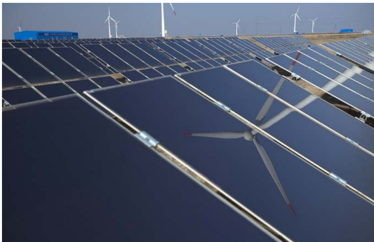
Dafeng Power Station is China's largest solar photovoltaic-wind hybrid power station, with 220MW of grid-connected capacity, of which 20 MW is solar PV. Located in Yancheng, Jiangsu province, it came into operation on December 31, 2010 and has 1,100 annual utilization hours. Every year it can generate 23 million KW-h of electricity, allowing it to save 7,000 tons of coal and 18,600 tons of carbon dioxide emissions. 11 Apr, 2011. © Greenpeace / Zhiyong Fu ▲
